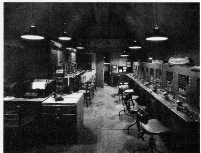
The telephone exchange in Casemate Level. Photo from English Heritage
